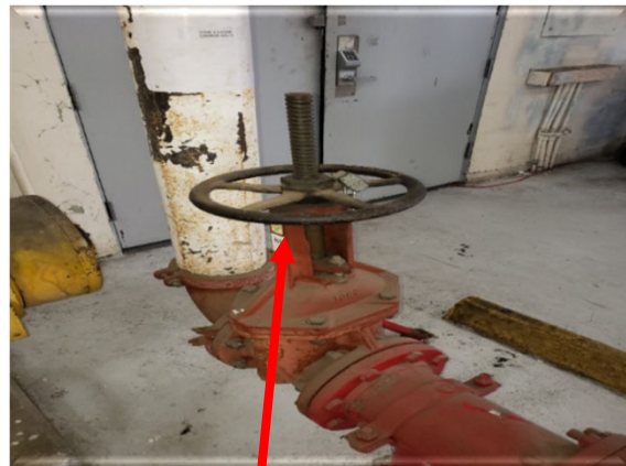
Manual Shut Off Control Valve (turn clockwise)
