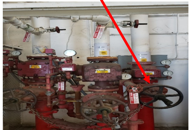
Manual Shut Off Control Valve (turn clockwise)
