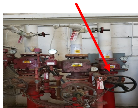
Manual Shut Off Control Valve (turn clockwise)
