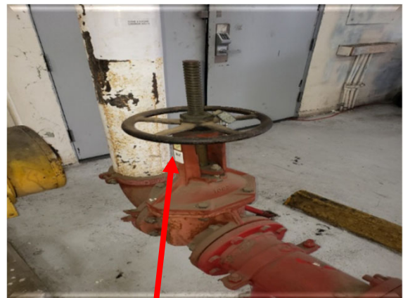
Manual Shut Off Control Valve (turn clockwise)
